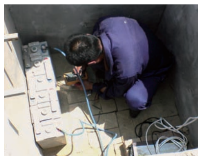
In Gansu, we installed power station batteries underground to reduce energy consumption
