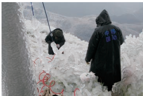
In Guangxi, we restored damaged lines caused by snowstorms
