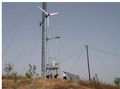
In Shaanxi, we introduced wind-solar hybrid power supply systems for base stations
