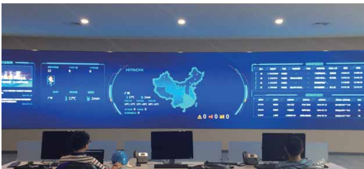
▲ IoT escalator monitoring platform
